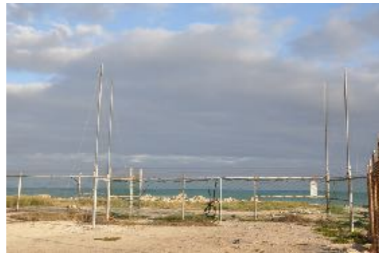
KAL HFR Tx antennas
