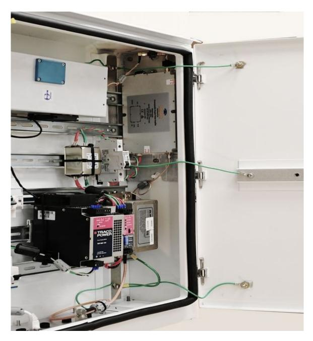
On the right wall: the power amplifier module and the low-pass filter.
